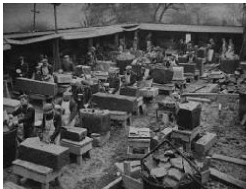
Stone masons repairing the Liverpool Cathedral after its bombing during World War II.
